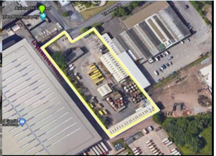
Figure 21: Li-ion battery recycling plant, Wolverhampton
