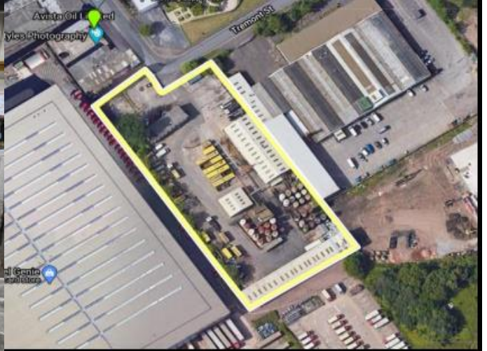
Figure 3: Li-ion battery recycling plant, Wolverhampton
